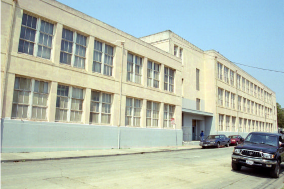
Figure 4: Classroom Building, exterior east wall
