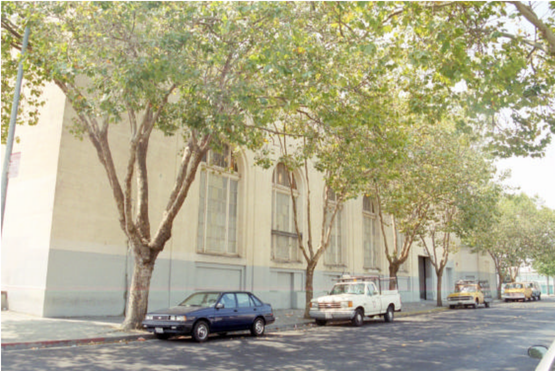
Figure 11: Auditorium Building, exterior north wall
