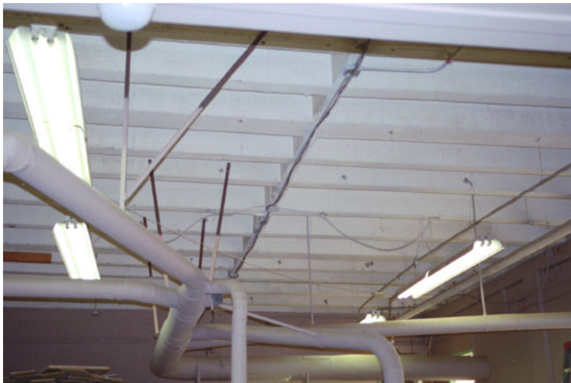
Figure 9: Classroom Building, interior exposed structure
