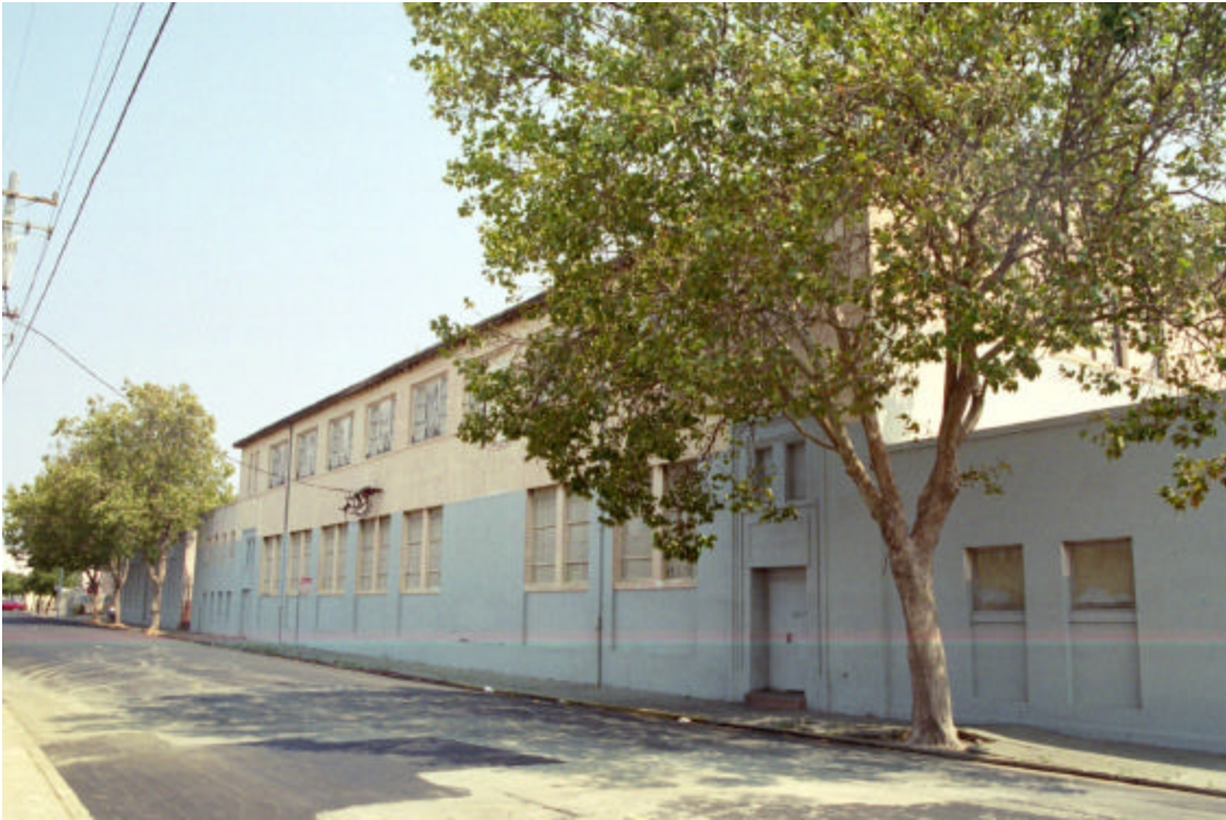
Figure 15: Gymnasium Building, exterior west wall
