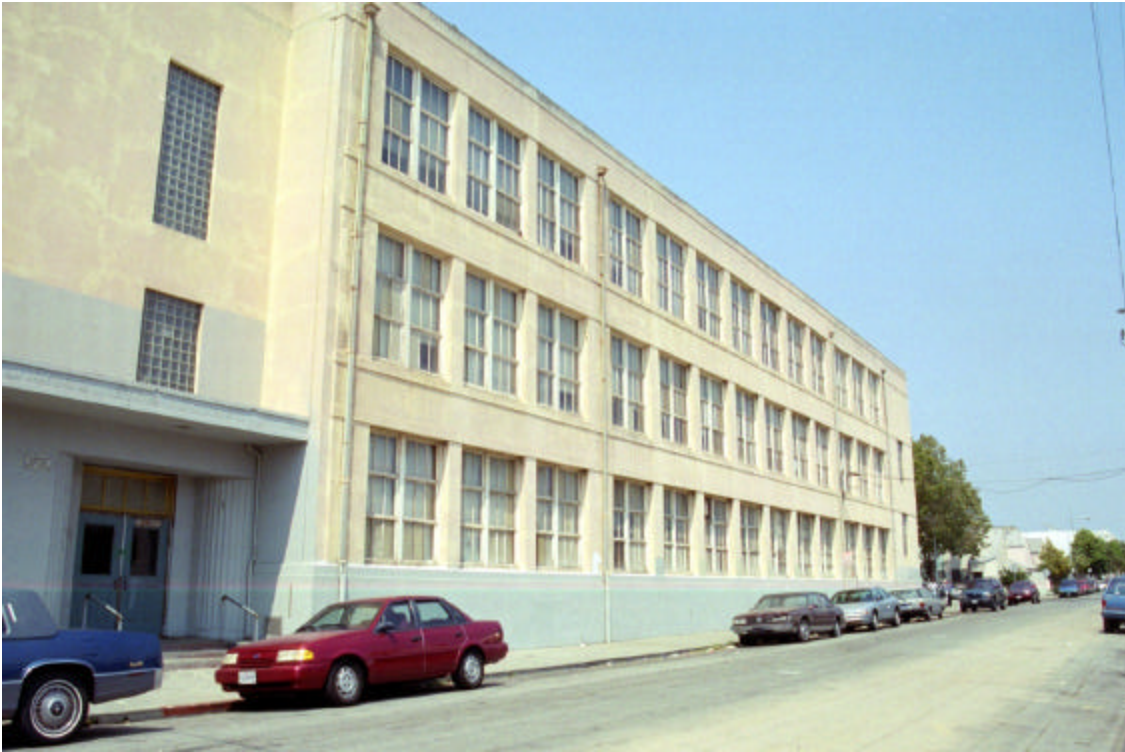
Figure 3: Classroom Building, exterior east wall
