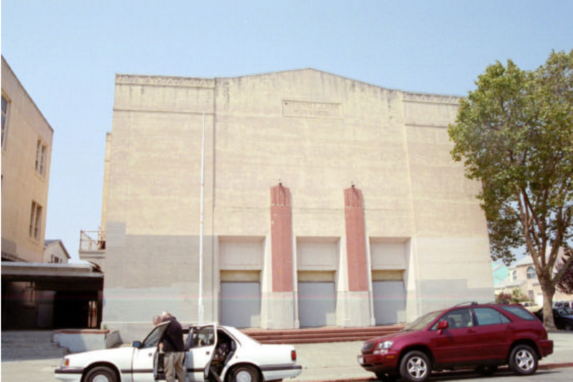
Figure 10: Auditorium Building, exterior east wall
