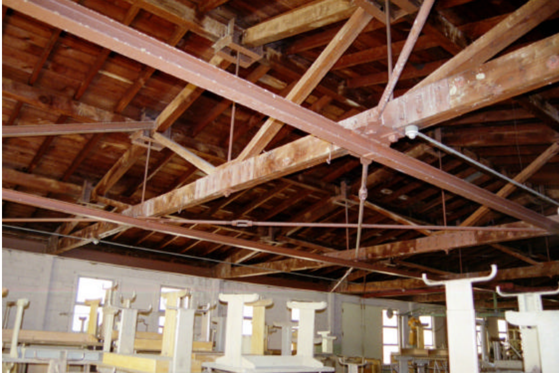
Figure 18: Gymnasium Building, interior exposed roof framing
