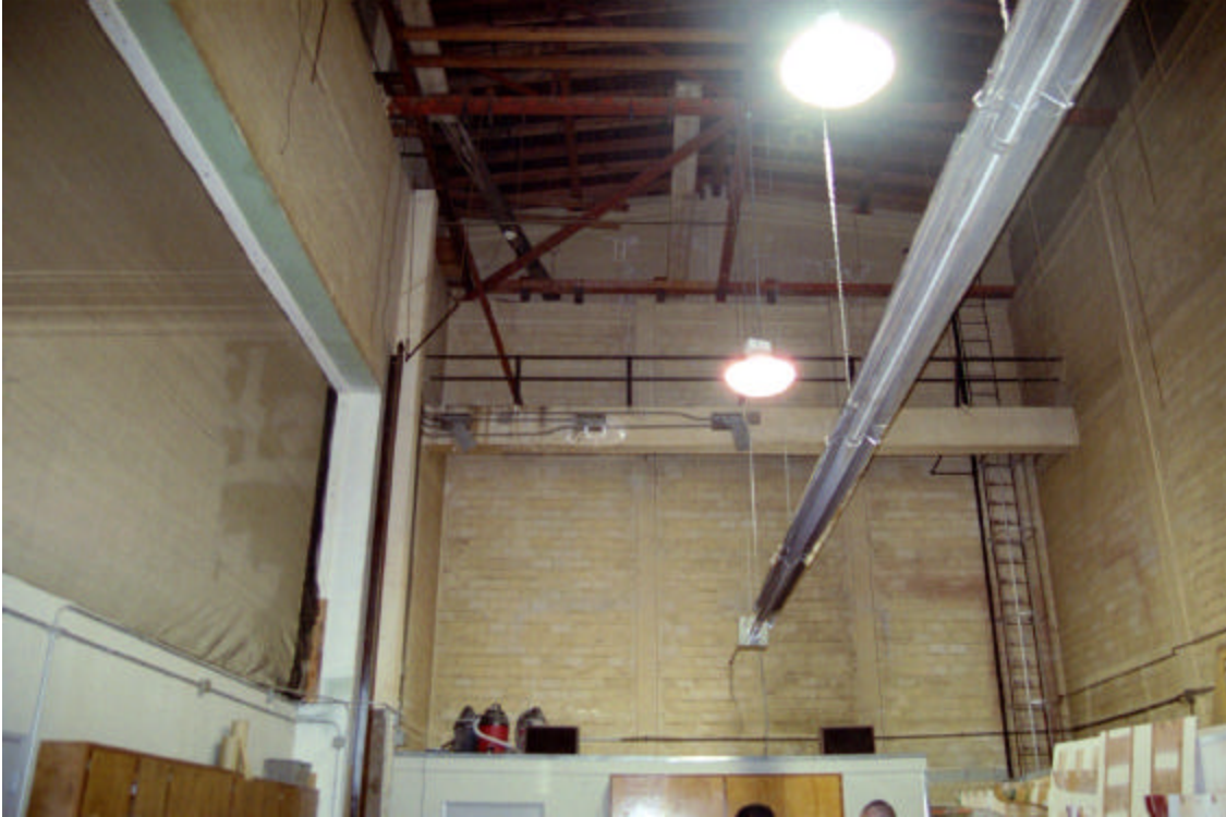
Figure 14: Auditorium Building, interior at former stage area
