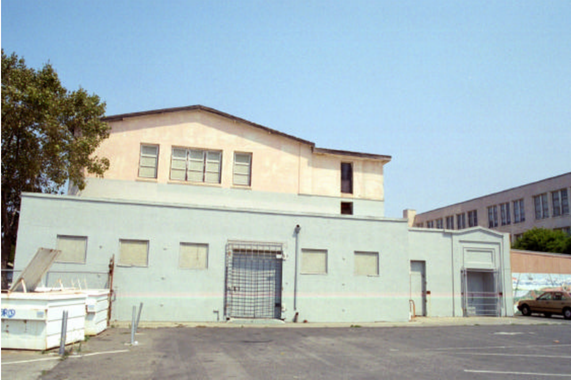
Figure 16: Gymnasium Building, exterior south wall
