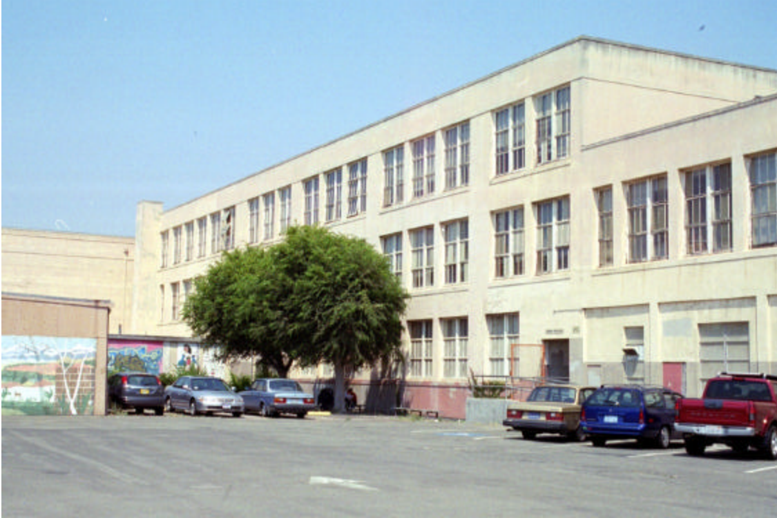
Figure 6: Classroom Building, exterior west wall
