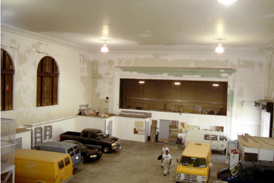
Figure 12: Auditorium Building, interior southwest corner
