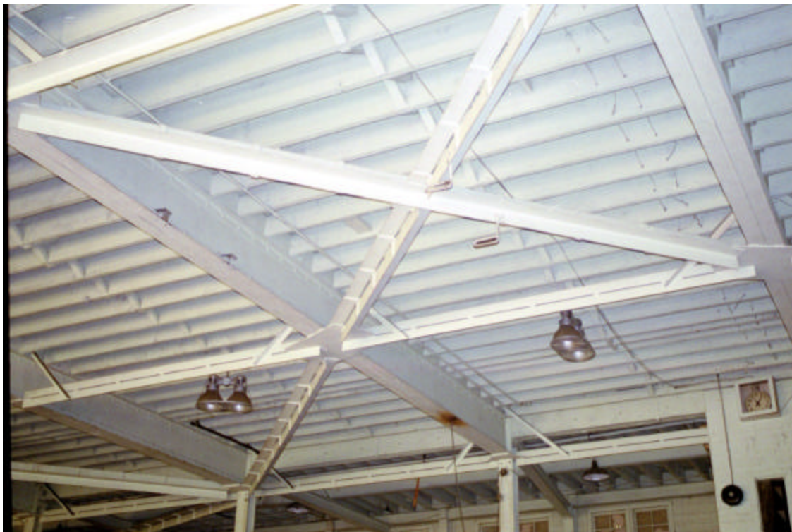
Figure 19: Gymnasium Building, interior exposed floor framing
