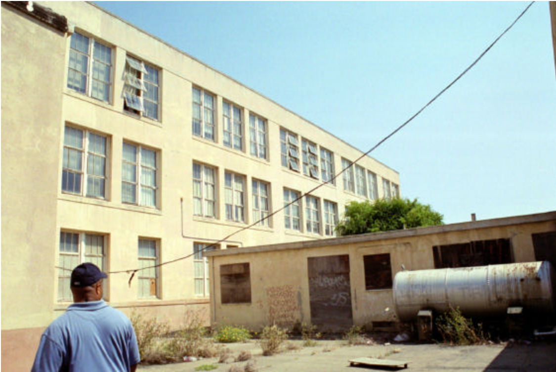
Figure 7: Classroom Building, exterior west wall
